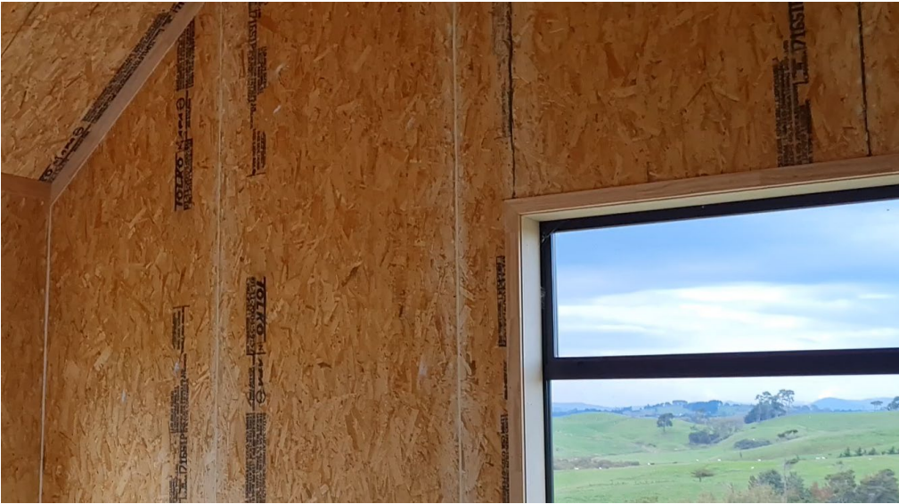
Figure 1 – Showing the interior of Formance SIP panels with typical millmarks
