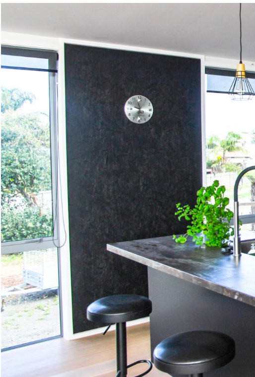
Figure 2 – Exposed Formance SIP showing the use of solid colour paint
